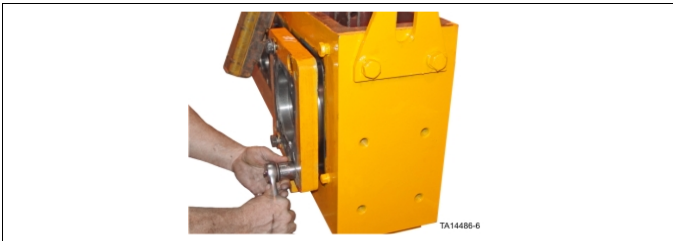
Figure 26. Installation of rear output bearing housing
