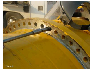
Cleaning paint and rust prior to torquing
